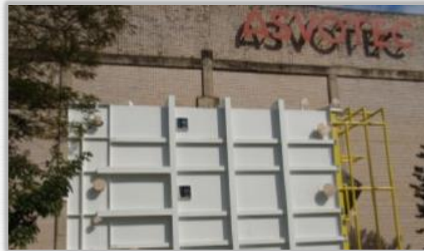
Diluent Deodulating Tank - OS: 23.966/2.006 2.500 X 3.002 X 6.251 mm - Weight: 7,4 Ton
